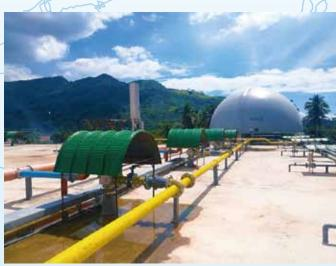
View from on top of the digester boxes: flare, pipeline and gas holder
