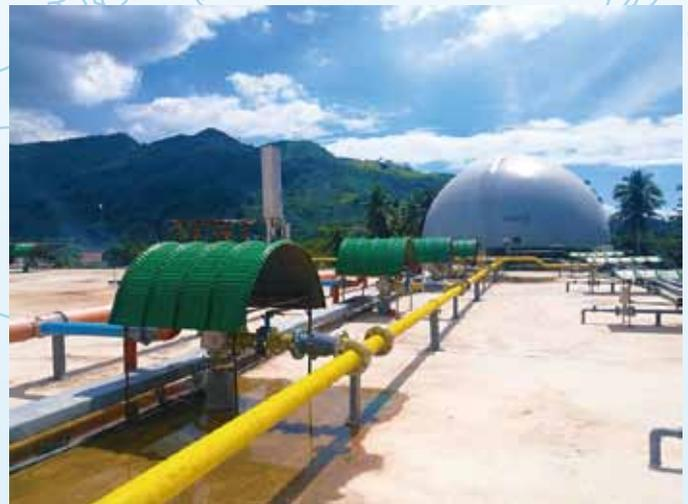
View from on top of the digester boxes: flare, pipeline and gas holder
