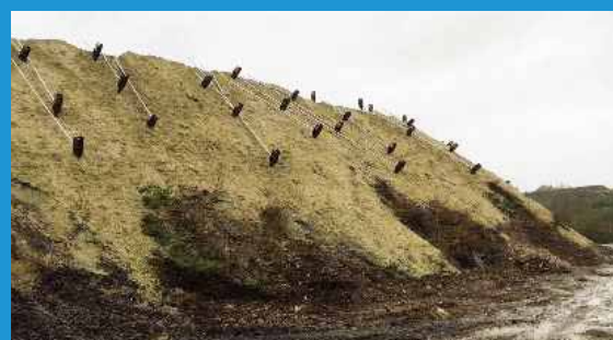
Aeration lances at the Remo landfill, Belgium
