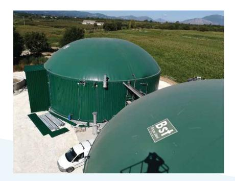
The resulting biogas is lighter than the substrate itself, and accumulates in a gas dome located directly above the substrate. The dome is constructed of flexible low pressure double membrane. Typically, more than half of the resulting gas is methane  $(CH_4)$ ; the rest is carbon dioxide  $(CO_2)$ .
