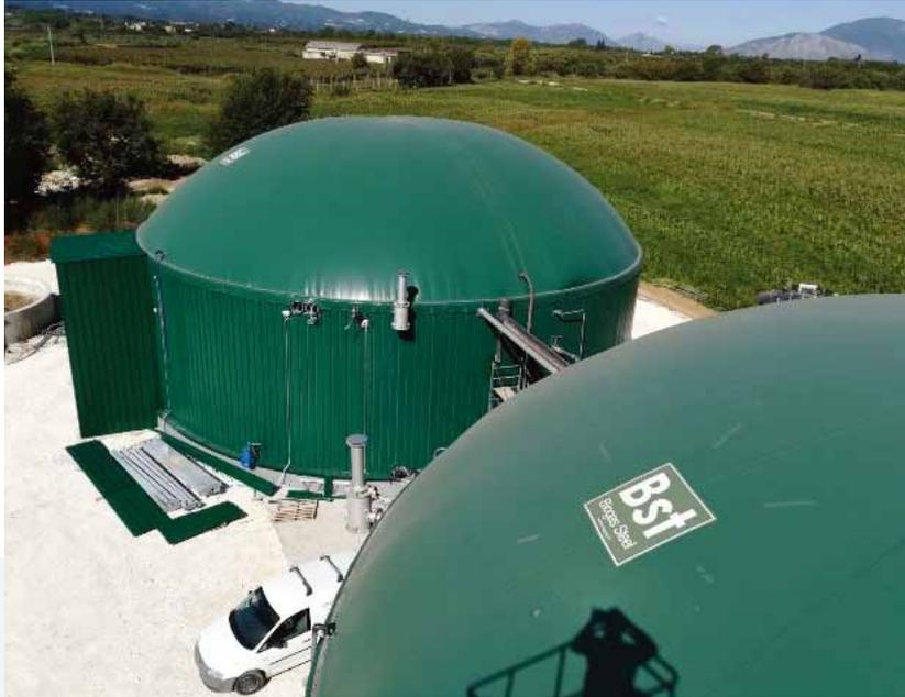
The resulting biogas is lighter than the substrate itself, and accumulates in a gas dome located directly above the substrate. The dome is constructed of flexible low pressure double membrane. Typically, more than half of the resulting gas is methane ( $\text{CH}_4$ ); the rest is carbon dioxide ( $\text{CO}_2$ ).
