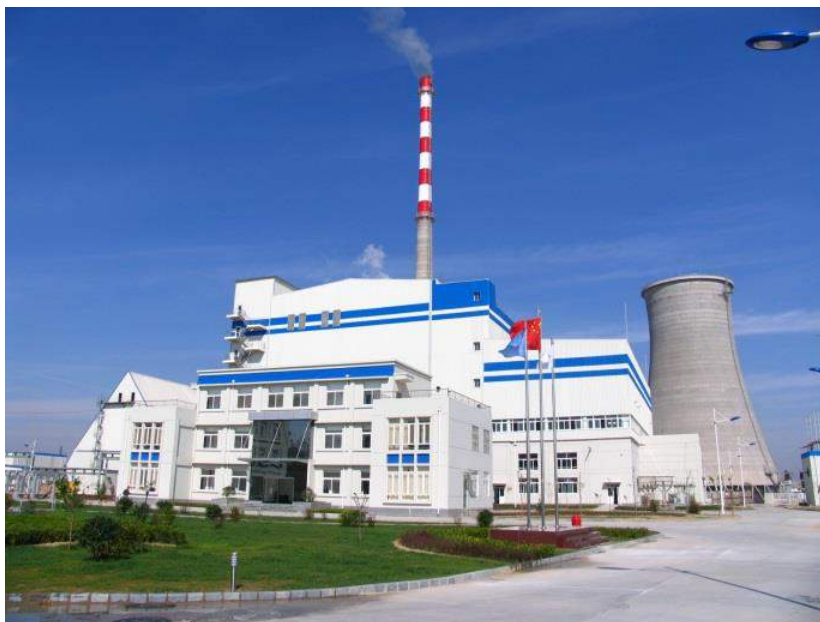
The first biomass power plant in China – DPCT/NBE Shanxian power plant
